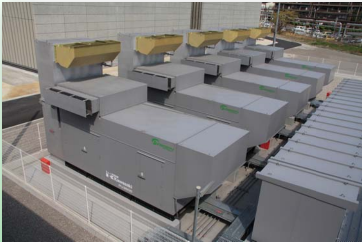
GPS3000 Light Weight High Power Density Back-up Units - Roof Mounted for Data Center
